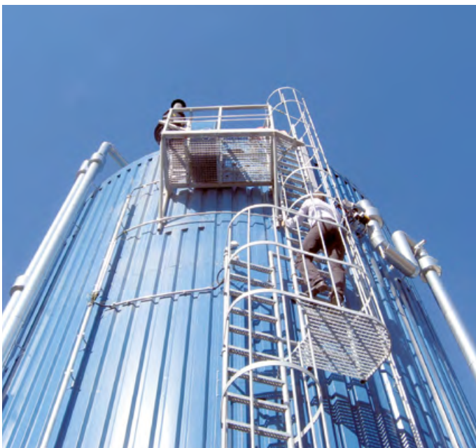
The sewage sludge is converted in a digestion tank from bacteria to biogas, which can then be used to generate power and heat.
